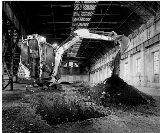
Fig. 14.7 Fraunhofer IOSB autonomous digger (Fraunhofer IOSB)
